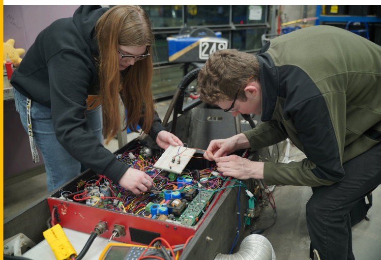
SEEN ABOVE: Electrical Team Member - Jessica Durham and Team Lead - Noah Bugden, inspecting wiring in the HV box.
